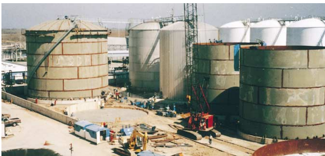
Work in progress to complete Bay 14 at Baytank.
