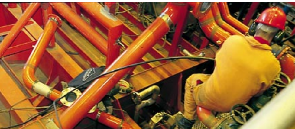
Connecting 20 km. of stainless steel piping.
