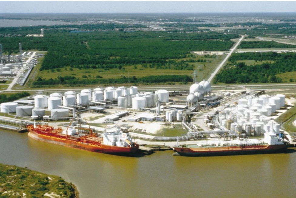
The tank terminal Baytank.
