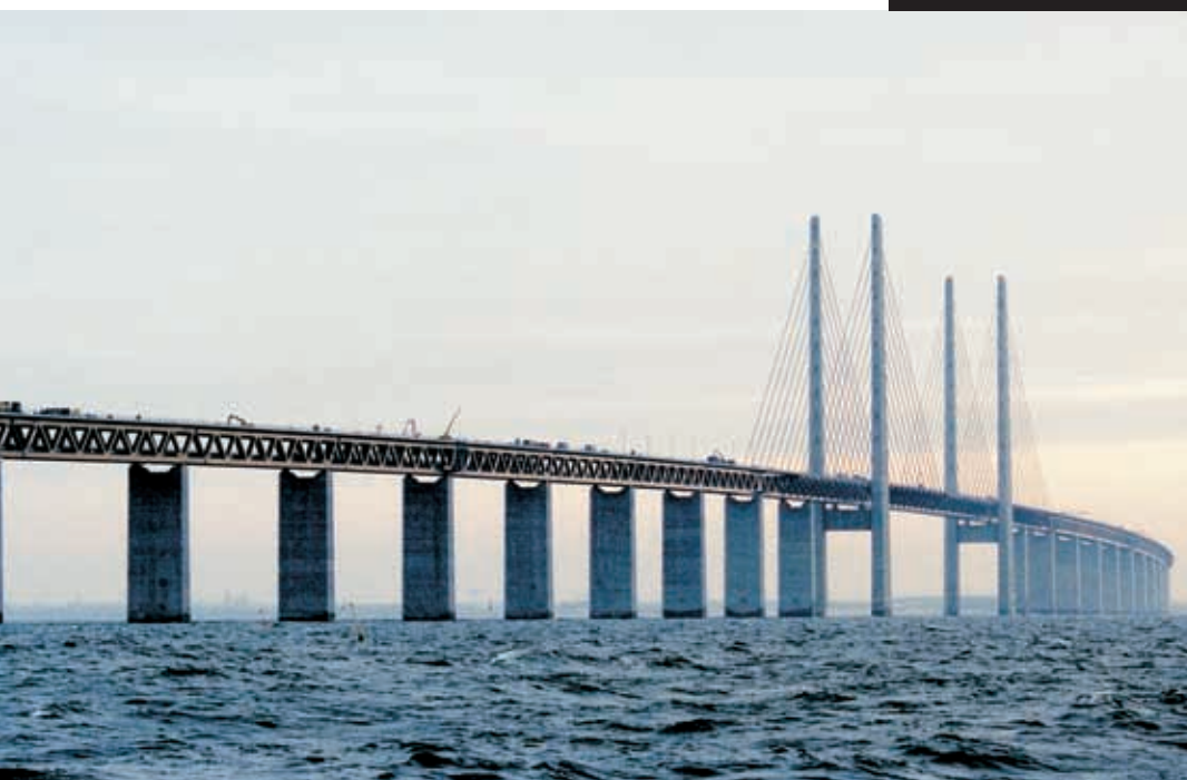
Elkem Microsilica® strengthens concrete in the Øresund bridge/tunnel project between Denmark and Sweden.
