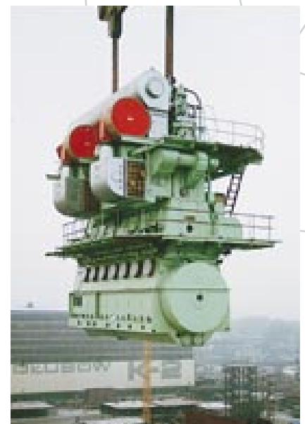
Lifting the main engine on board.
