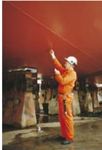
Members of the Site team checking paint thickness and installation details.
