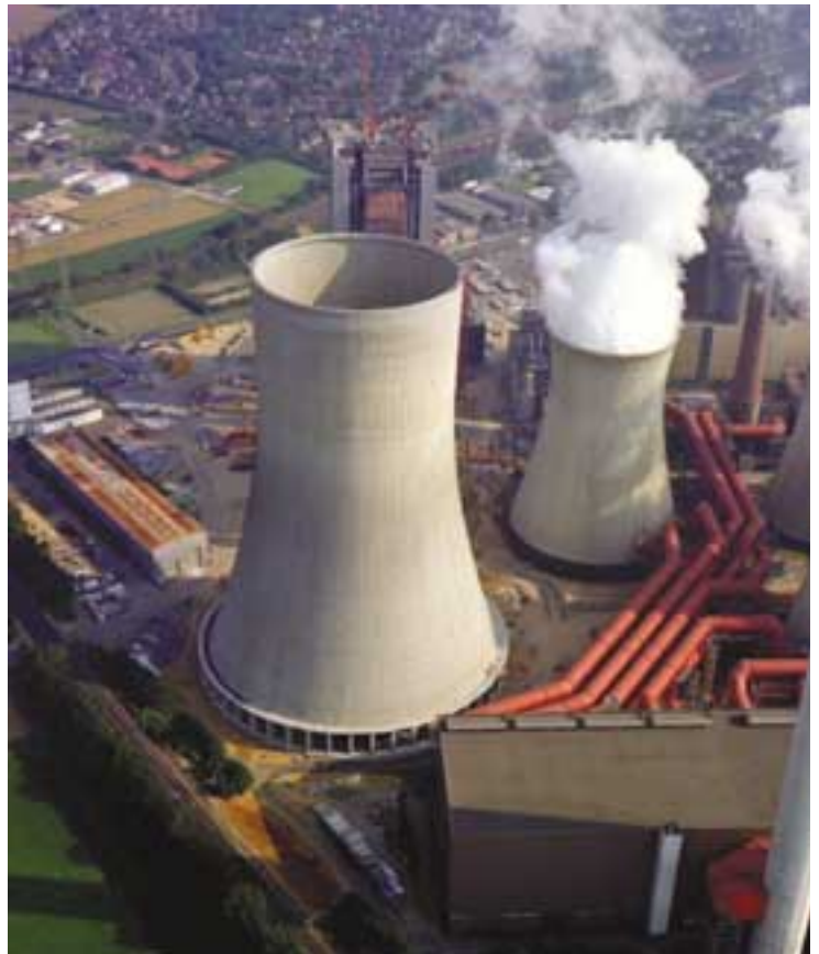
FESIL Microsilica slurry is used in about 21,000 m 3 concrete for a cooling tower in a coal fired power plant in Germany. The cooling tower was built during 1999-2000, and has a height of 200 m. Bottom diameter is 136 m, top diameter is 87 m. The cooling tower also works as chimney, where there is some sulphuric acid in the flue gases. The reason for using microsilica in the concrete was to achieve a high strength concrete, resisting against acid attack. The microsilica slurry was delivered from FESIL's customer MC Bauchemie.
