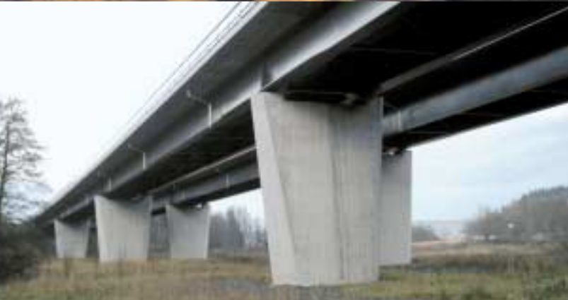
At Gleborg north of Uddevalla, Veidekke has built two double bridges, which help to direct the traffic away from the built-up area and make the E6 highway and the road to Liseberg both quicker and safer.
