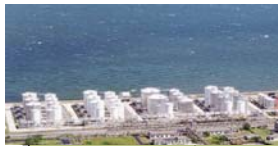
OTD, Dalian 60,000 cbm – 35 tanks
