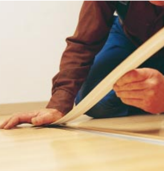
Remel™, Perstorp's fiber-glass reinforced melamine plastic, was launched successfully within such sectors as telecommunications, white goods and transport, as well as in the construction industry, where pattern-adapted Remel™ moldings are included in Perstorp's flooring range.
