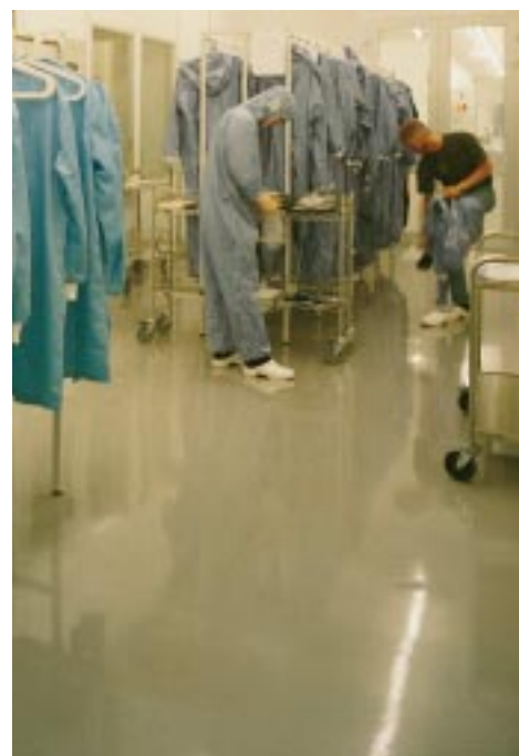
Perstorp's sales of seamless industrial surfaces are increasing sharply, particularly in the electronic, food and pharmaceuticals industries, as a result of escalating hygienic and environmental demands.
