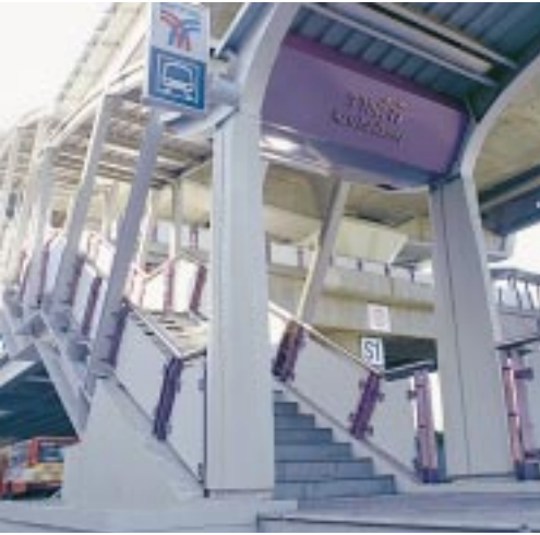
In Bangkok, Thailand, Perstorp Surface Materials is delivering a broad spectrum of surface materials solutions to 23 stations in BTS, the city's new public transport system.
