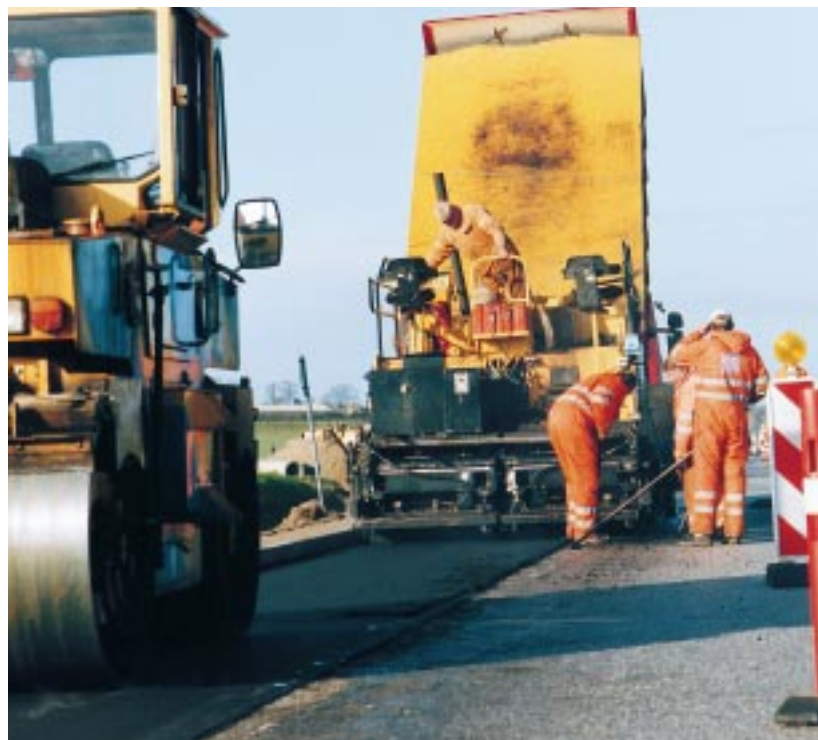
Road surfacing with asphalt.
