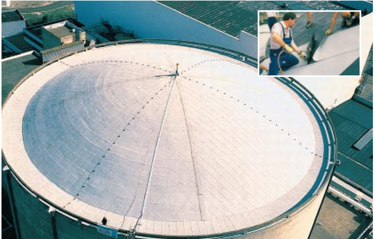
Icopal roofing felt was used to renovate the roof at the Tihange nuclear power station in Belgium.
