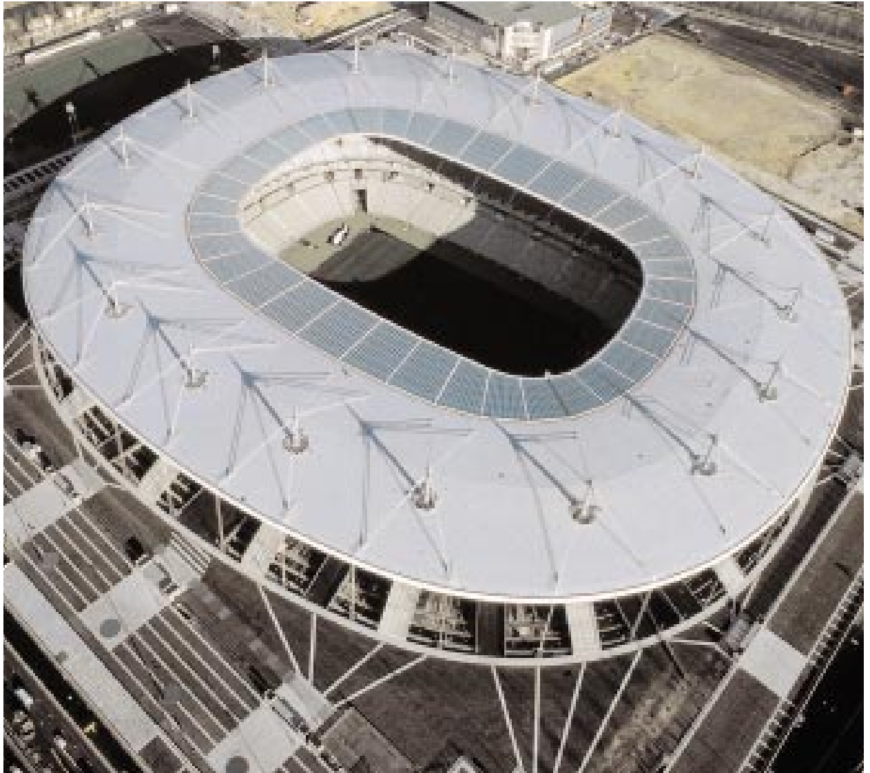
Siplast S.A. has delivered 20,000 square meters of Parafor Ponts, Paraforix and Teranap for the annexe stadium, a training area close to the new "Stade de France".
