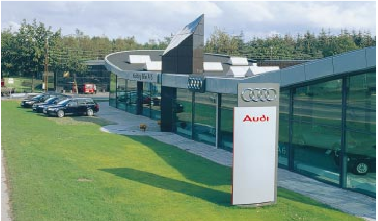
Icopal was given the roofing contract for Kolding Biler's new car showroom.
