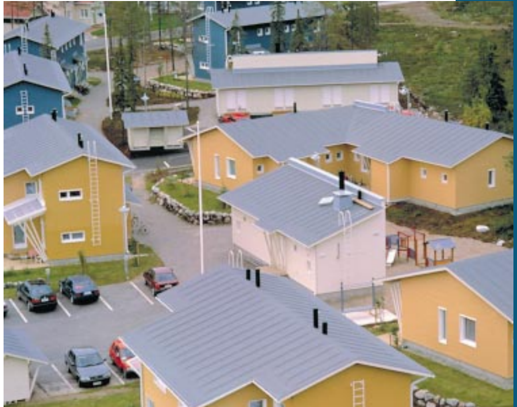
Profiled roofing on 7,000 m 2 of roof at a housing exhibition in Rovaniemi, Finland.
