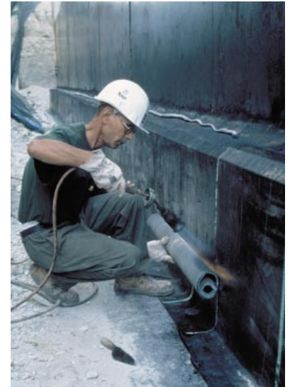
Welding bitumen membrane.
