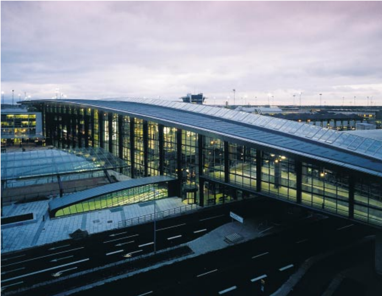
The new international terminal at Copenhagen International Airport has been covered with Icopal roofing felt.
