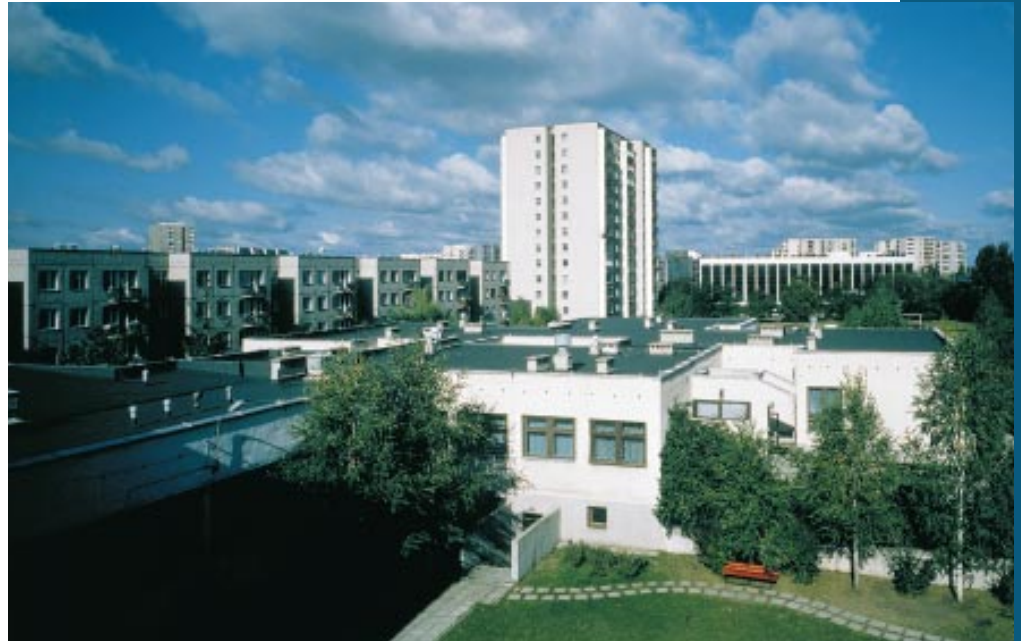
Schools and other centres for children in the municipality of Vrsynow, in Poland have Icopal felts on their roofs.
