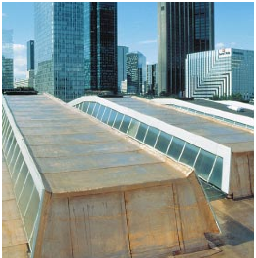
The roof of the French Nautical Club's building at Neuilly has been covered with a copper-surfaced felt.
