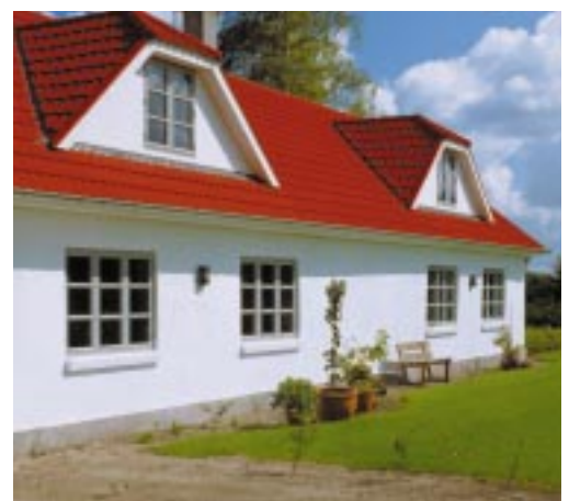
This farm's roof has been completely renovated with red Decra.
