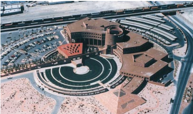
The roof of Clark County's municipal building in Nevada has been covered with Siplast's lightweight insulation system and surfaced with Paradiene roofing felt.
