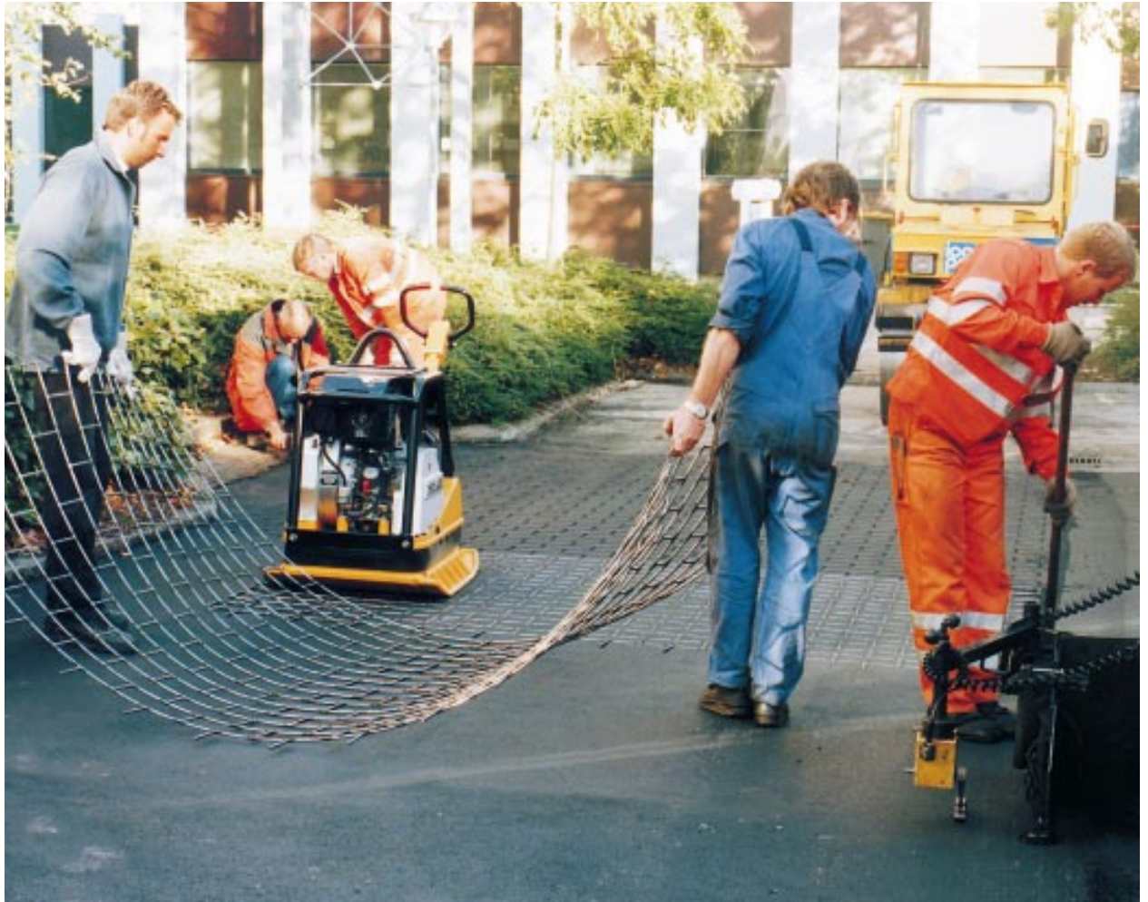
Icopal's Roads Division has bought the rights to the American product "Street Print", which is used to pattern asphalt.
