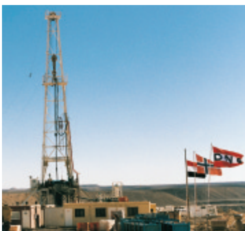
DNO drilling rig on Tasour Field in Block 32 - Yemen
