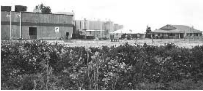
Borregaard LignoTech has established strict environmental requirements at its new plant for lignin-based products at Mt. Vernon, south of Seattle, USA. As the entire process is closed, chemicals are recycled in such a way that the plant has no discharges to water.
