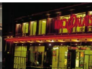
Kinopalatsi, Sandrew Metronome's new 10-screen cinema complex in Helsinki, had its first full year of operations in 1999.
