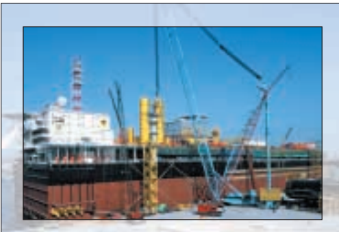
GIRASSOL FPSO UNDER CONSTRUCTION
