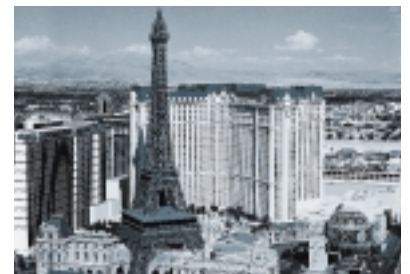
Also in the Paris Hotel, Las Vegas / USA, Belimo actuators and valves are in operation.
