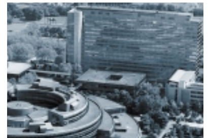
Retrofit of heating and cooling water circuits with Belimo products in the high-rise on the ZDF television premises in Mainz / Germany.
