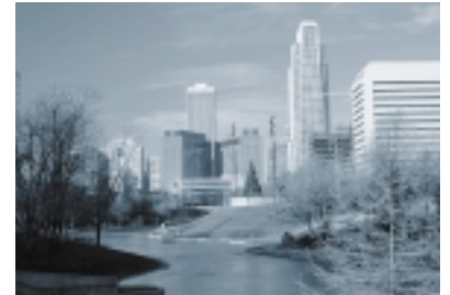
Center of Omaha, Nebraska / USA: All buildings on the photo are equipped with Belimo actuators.
