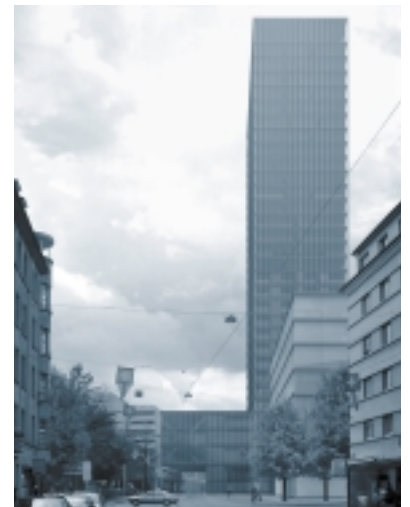
The new trade fair tower in Basel / Switzerland with fire protection and smoke extraction solutions from Belimo.
