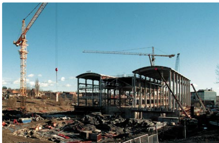
The new printing plant in Nydalen estimated at NOK 1,4 billion.
